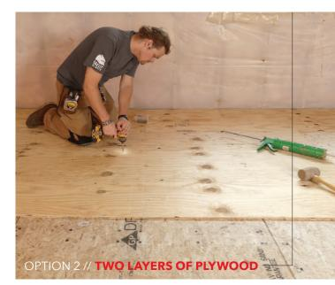
Another popular way of creating a wood subfloor is to install two layers of plywood—with the top layer laid out perpendicular to the bottom—and let them float over the vapor retarder or the vapor retarder and foam. Applying adhesive between the layers in addition to the screws will ensure a solid bond. While more time will be spent hauling, cutting, and positioning the plywood, floating two layers of plywood eliminates the need for masonry fasteners and helps mitigate issues with warped plywood.
